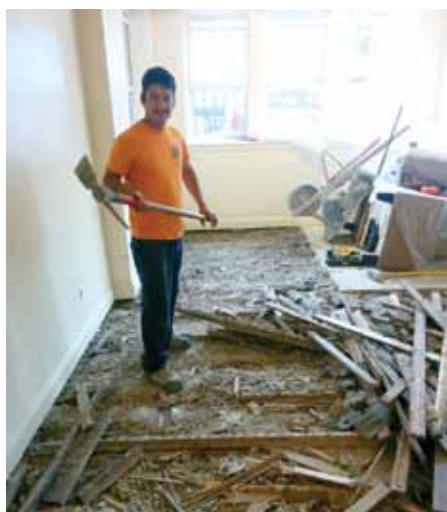
Project Fierce House renovations.
